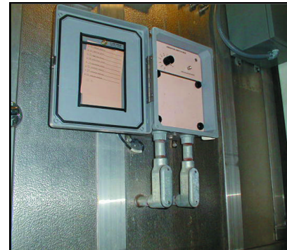
Figure 6 - Another option is to mount a conduit fitting to the side of the housing and run the wires through conduit.
