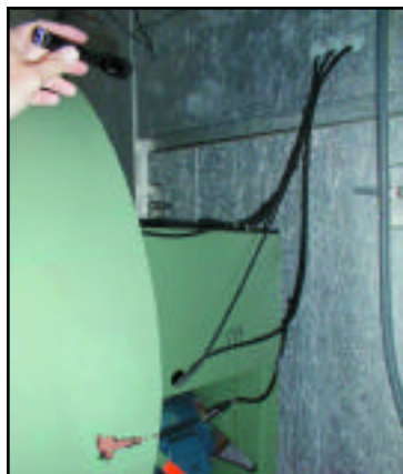
Figure 4 - Cables should be tied together so they cannot be damaged by rotating equipment, and should exit from the air handler unit in a centralized location.
