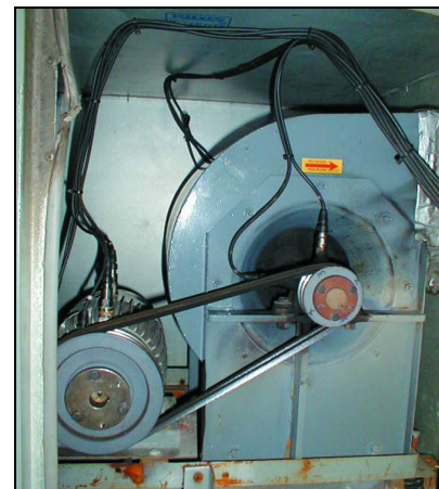
Figure 2 - The air handling units have fairly typical rotating elements, composed of two shafts supported by rolling element bearings, connected by a sheave-and-belt combination.
