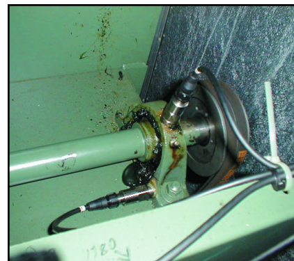
Figure 3 - To provide the optimum vibration transfer between the machine surface and the accelerometer, a mounting system that utilizes the full frequency span of the accelerometer needed to be considered.
