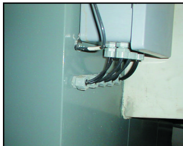
Figure 5 - One option used for this was to drill a hole in the side of the housing for installation of a cord grip and then seal it upon installation with silicone RTV.
